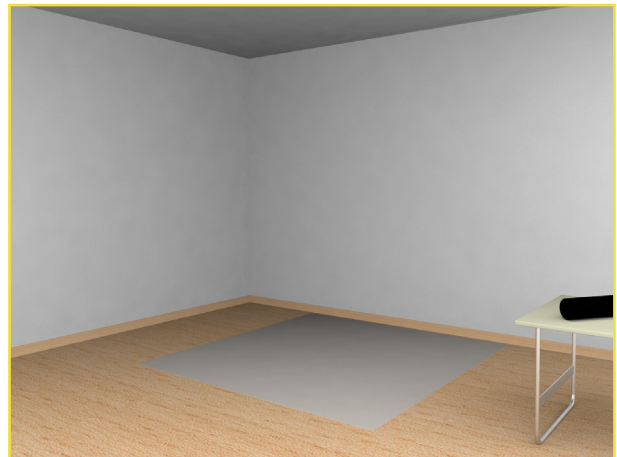
Fig.21: Laying out the underlay
