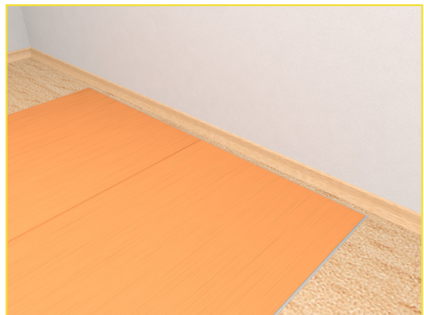
Fig.22: Laying out the screen material
